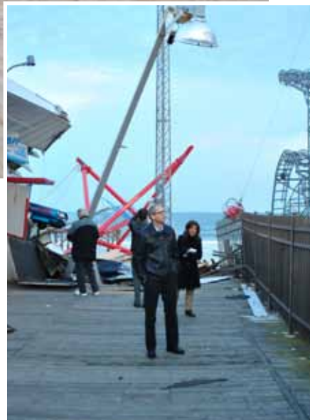
BELOW: Kenneth Schwartz, dean of the Tulane School of Architecture, joined the NJIT faculty members assessing damage caused by Hurricane Sandy at the New Jersey shore.
