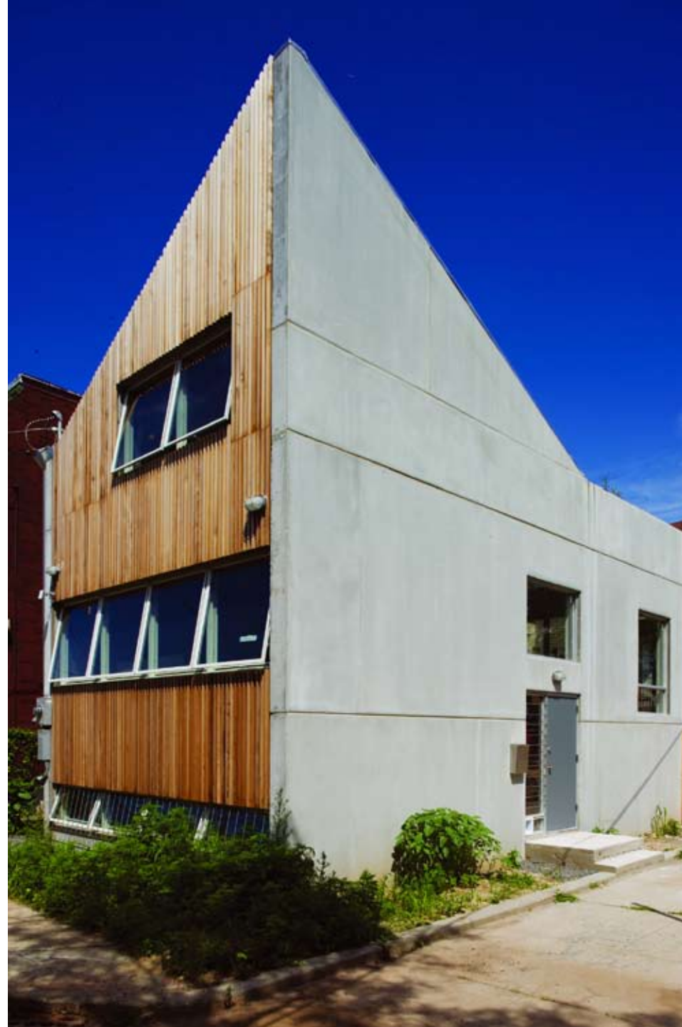
The PREtTyFAB house in Jersey City – at the leading edge of high-performance design
