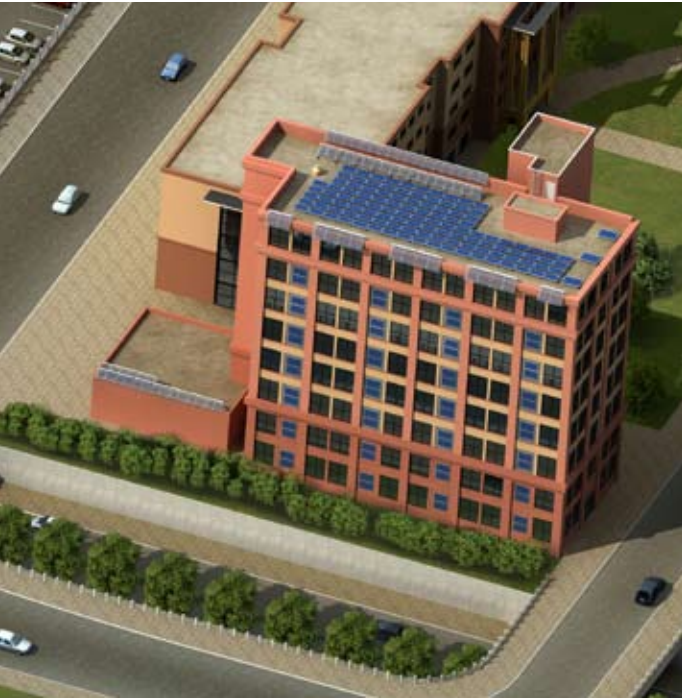
This architectural rendering shows the solar heating panels and photovoltaic cells that will be installed on the roof of Oak Hall.
