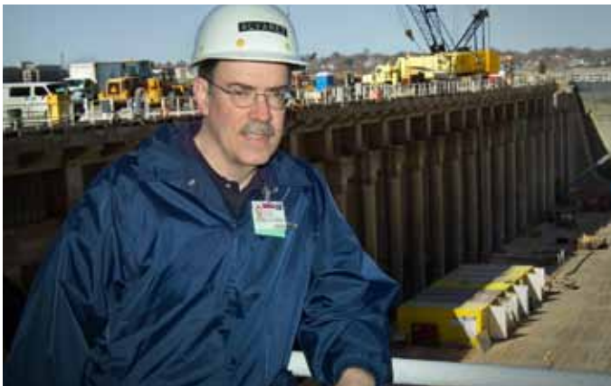
Austin Alvarez at Electric Boat Corporation's Graving Dock 3 before major reconstruction.
