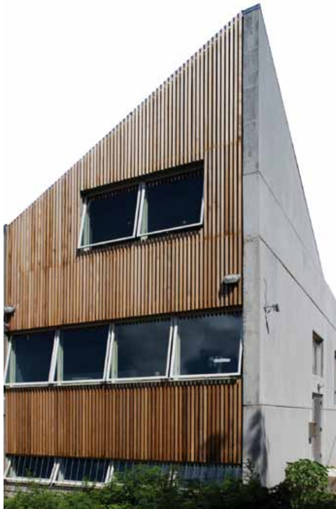
PHOTO: COURTESY GRO ARCHITECTS
