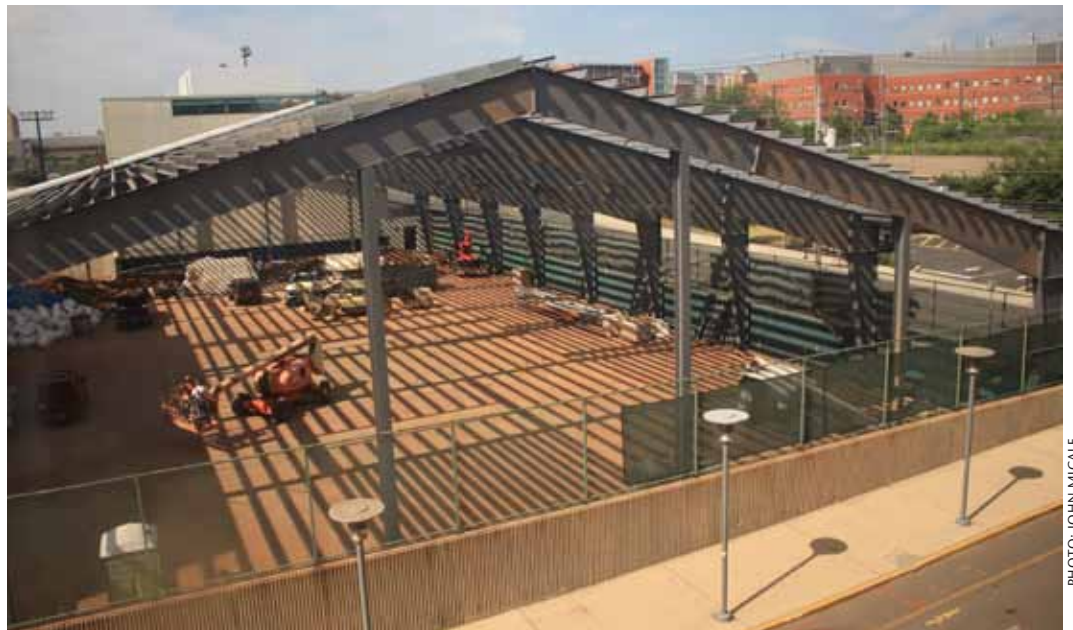
The Naimoli Family Recreation Center under construction
